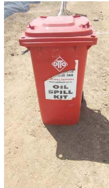
4. Tier 1 level spill kit at loading ramp
